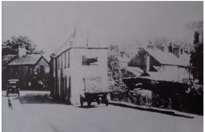
The Horseshoe Inn, Croston – demolished in the 1930’s for road widening.
